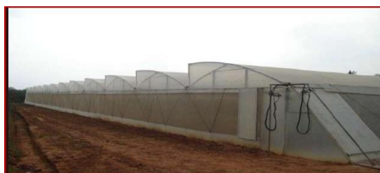
Fig. 17.5 Saw tooth type greenhouse
