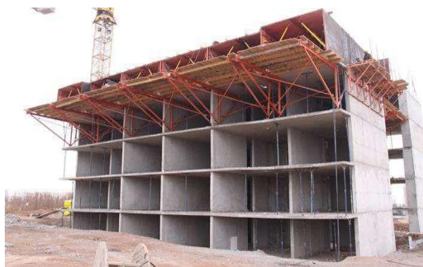
Fig. 14.4 Tunnel Formwork System
