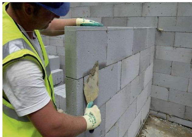
Fig. 14.6 Thin Joint Masonry Technique
