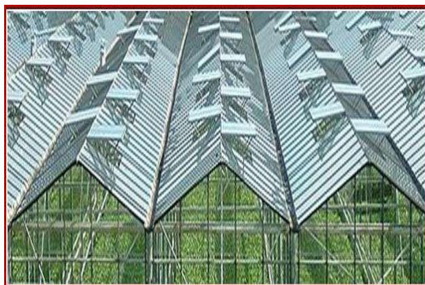
Fig. 17.4 Ridge and furrow type greenhouse
